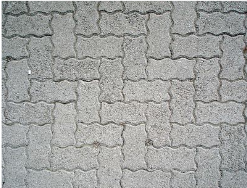
FIGURE 5. Second Brick Tiling.
